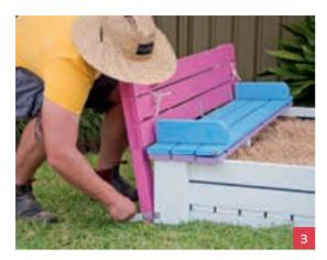
**3. By fitting a hasp and staple** to each side of the sandpit, you can use a padlock to secure it in an open or closed position.
