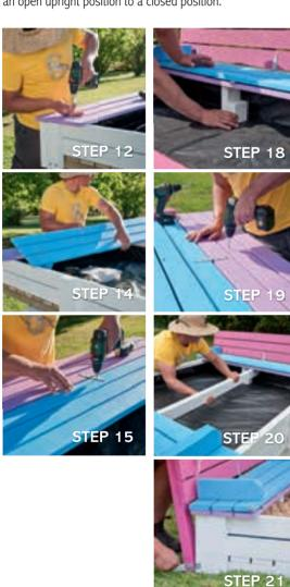
reeded-face down, centred to short side of frame and flush with outside of corner battens. Predrill, then screw-fix decking to sides. Repeat to fix 3 remaining purple lid decking lengths to other side.
